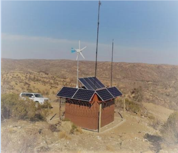
Figure 2: Embassy Windhoek's solar-powered repeater (Source: OIG).
