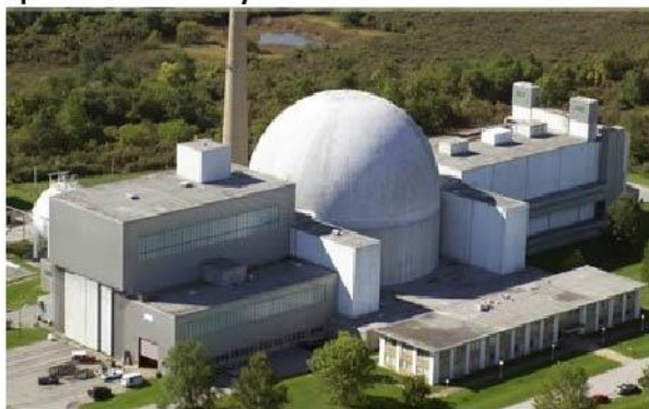
Space Power Facility
