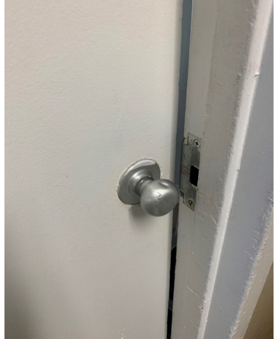
Photograph 1 (left): Exit door obstructed by boxes. Photograph 2 (right): Corridor door would not latch or seal.
