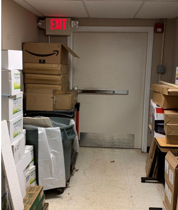
Photograph 1 (left): Exit door obstructed by boxes. Photograph 2 (right): Corridor door would not latch or seal.
