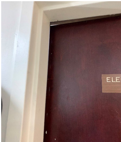
Photograph 3 (left): Self-closing door would not fully seal. Photograph 4 (center): Electrical room smoke barrier would not seal. Photograph 5 (right): Missing and damaged ceiling tiles.
