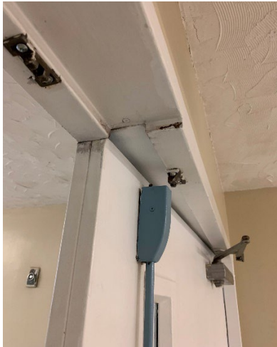
Photograph 3 (left): Self-closing door would not fully seal. Photograph 4 (center): Electrical room smoke barrier would not seal. Photograph 5 (right): Missing and damaged ceiling tiles.
