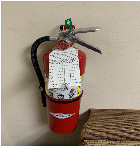
Photograph 6 (left): Fire extinguisher did not have monthly inspections.
