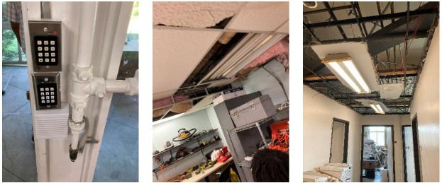
**Photograph 6 (left):** This emergency exit required a code for exit. **Photographs 7 and 8 (middle and right):** Ceiling tiles were missing or damaged.
