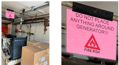
**Photograph 12 (left):** Items kept around the generator posed a fire risk. **Photograph 13 (right):** A sign above the generator shown in Photgraph 12 warns about the fire risk and tells people not to place anything around the generator.
