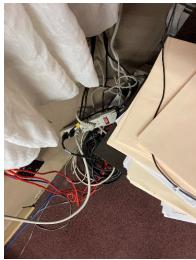
Photograph 19: Electrical wiring was "daisy chained."
