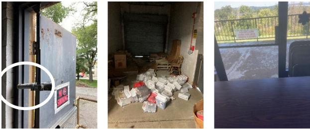
**Photograph 1 (left):** This exit door had a broken self-closing device, which prevented the door from closing automatically. **Photograph 2 (middle):** Biohazard materials were left on the floor and impeded the exit. Used biohazard materials were outside of their containers and posed a potential risk to people attempting to exit. **Photograph 3 (right):** This table was blocking an emergency exit.
