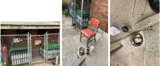
**Photographs 16, 17, and 18:** A smoking area was a few feet from an oxygen tank storage area with a "no smoking" sign. These oxygen tanks were also exposed to changing weather conditions.
