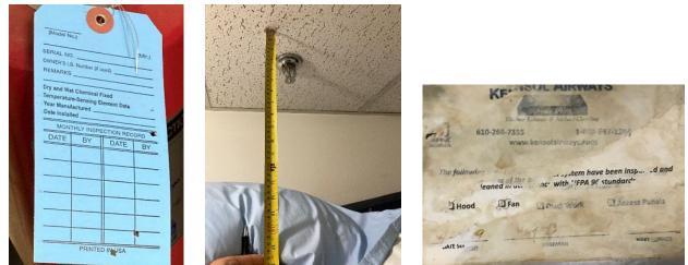
**Photograph 9 (left):** This fire extinguisher did not have any recorded monthly inspections. **Photograph 10 (middle):** This sprinkler head was obstructed by stored items; an 18-inch clearance is required for all sprinklers. **Photograph 11 (right):** As indicated by this inspection tag, the most recent kitchen hood inspection was in 2019, 2 years prior to our audit and with no next service date scheduled.
