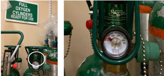
**Photograph 14 (left):** Empty oxygen cylinders were left in the "full oxygen cylinders" area. **Photograph 15 (right):** This close-up of the oxygen cylinder gauge from Photograph 14 shows that the gauge indicated that the oxygen cylinder was empty.
