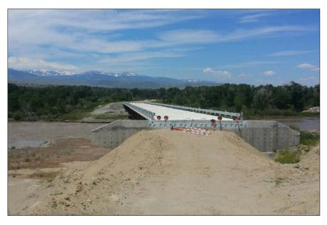
Figure 1. The Lenore Bridge project has not been completed, as the approaches still have not been constructed. Source: OIG.
