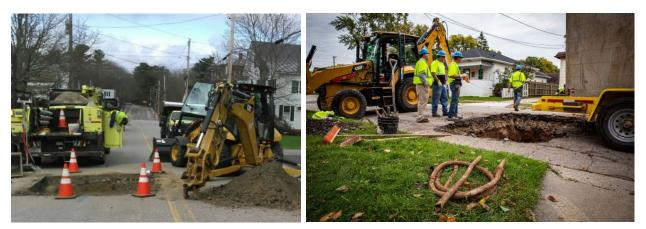
Construction work involving drinking water lead service line replacement. (EPA images)
