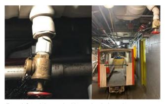
From left to right: cracked low point drain; train passenger cart. (U.S. Navy photos)
