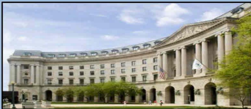
EPA headquarters in Washington, D.C. (EPA image)
