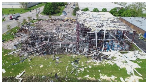
The CSB investigated an explosion and fire at the AB Specialty Silicones facility in Waukegan, Illinois. (CSB photo)
