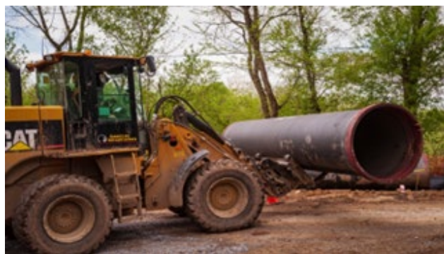
Water main installation in Frederick, Maryland. (EPA image)
