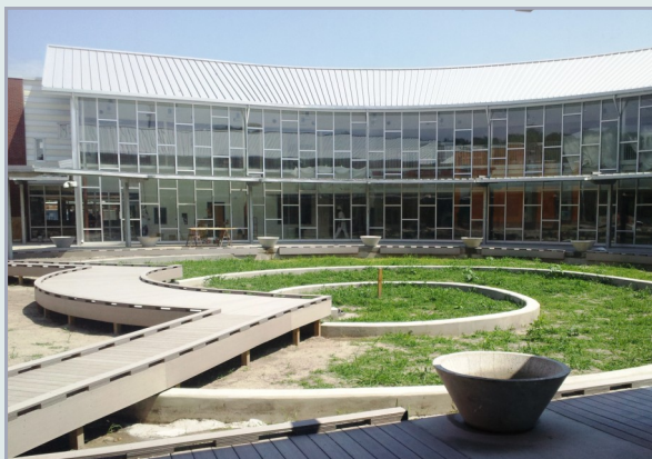
Source: OIG photo
