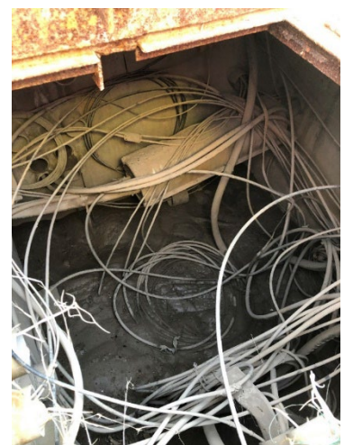
Figure 2: Cable laying directly on false ceiling (Source: OIG).
