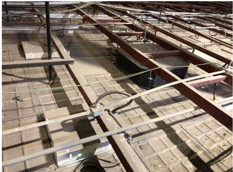
Figure 2: Cable laying directly on false ceiling (Source: OIG).
