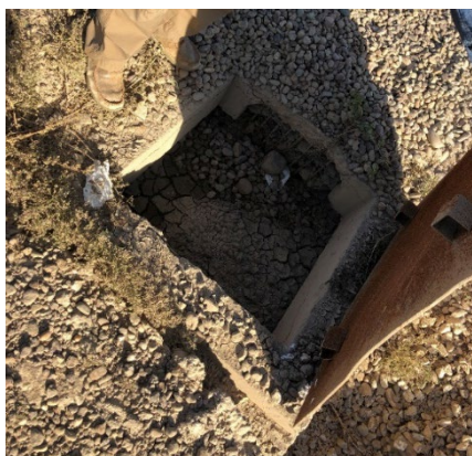
Figures 3, 4, and 5: Cable manholes filled with mud (Source: OIG).
