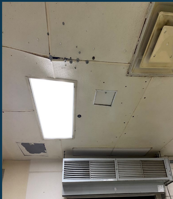
Left, Food Service Area Ceiling Panels Warped Due to Water Damage, Riveted Together to Maintain Overhead Cover. Right, Water Damage Rendered This Section of the Food Service Area Unusable.
