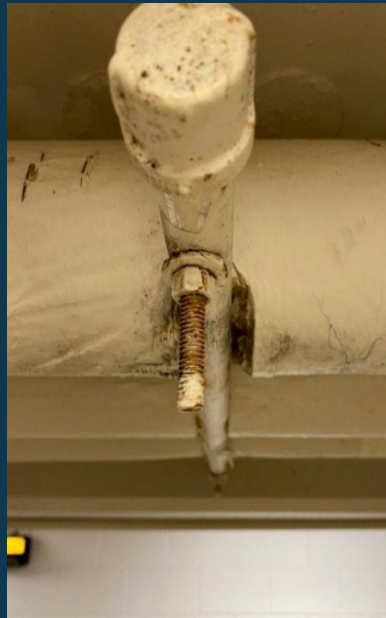
Left and Center, Bolt Attached to Overhead Pipe Close to an Inmate Bed, Right, Inmate-Fashioned Protective Covering on the Bolt
