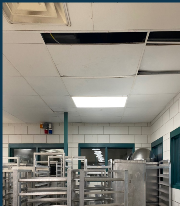
Left, Food Service Area Ceiling Panels Warped Due to Water Damage, Riveted Together to Maintain Overhead Cover. Right, Water Damage Rendered This Section of the Food Service Area Unusable.
