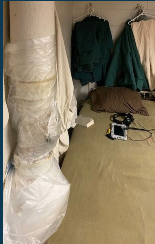
Condition of Pipes and Their Proximity to Inmate Beds in a Basement Housing Floor
