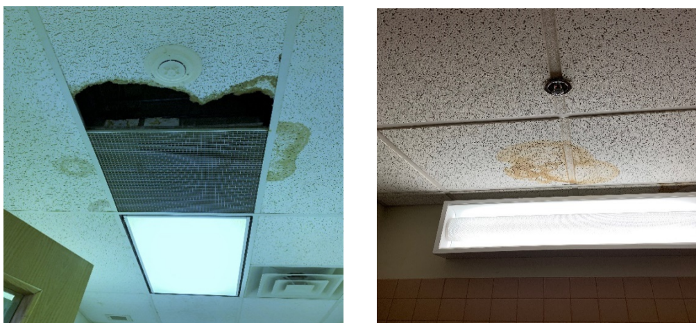
Figure 3: Ceiling Tile Damage at the Middle School (left) and Elementary School (right)
