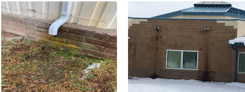
Figure 5: Downspout Draining Straight Down to the Foundation of the Administration Building (left) and Missing Downspouts at the Dormitory (right)
