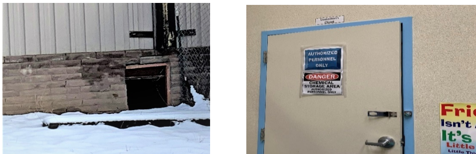
Figure 8: Unsafe Access to a Crawlspace at the FACE Portable Building and an Unlocked Custodian Closet at the Elementary School
