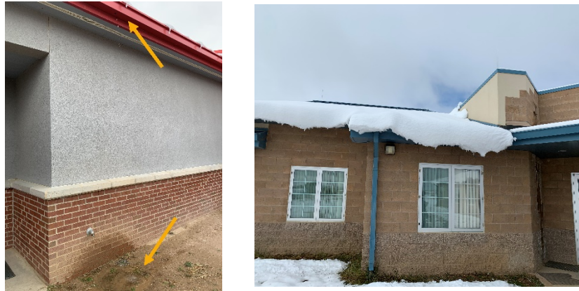
Figure 4: Hole in the Gutter at the Elementary School (left) and Snow on the Gutters of the Dormitory (right)
