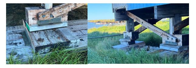
This foundation is unstable due to permafrost degradation. Blocks are placed under the original foundation to help stabilize the structure.
