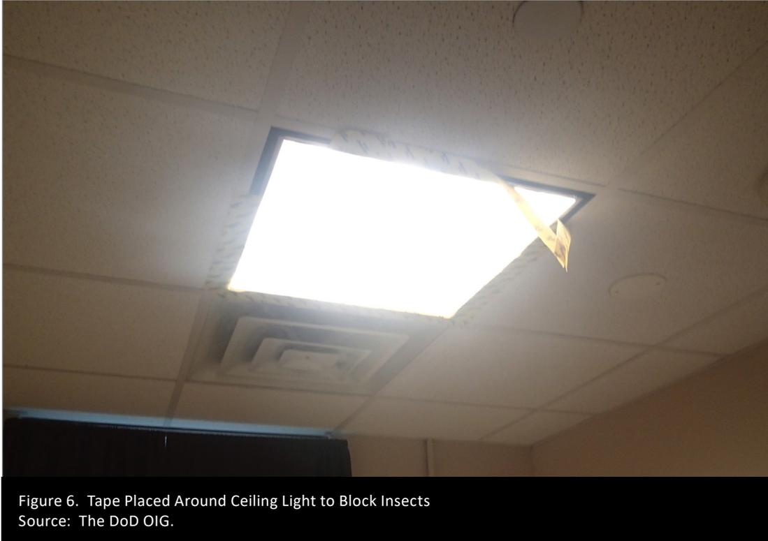
Figure 6. Tape Placed Around Ceiling Light to Block Insects
