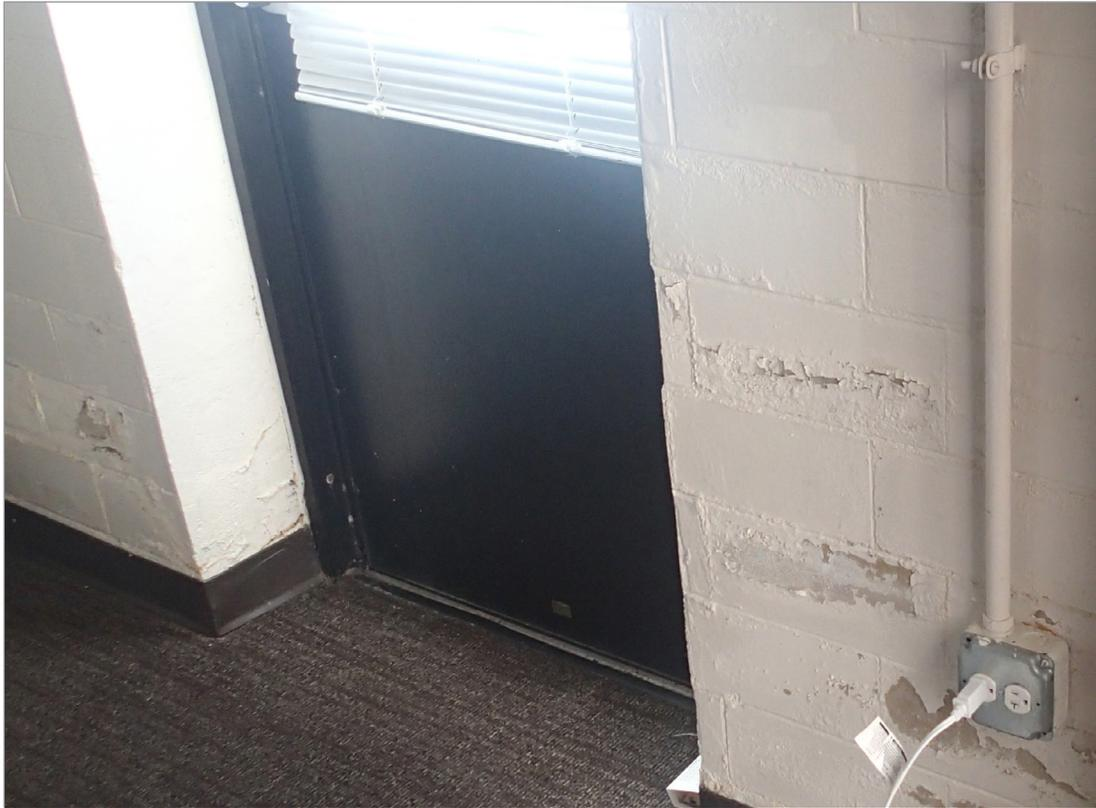
Figure 7. Peeling Wall Paint in Room 121
