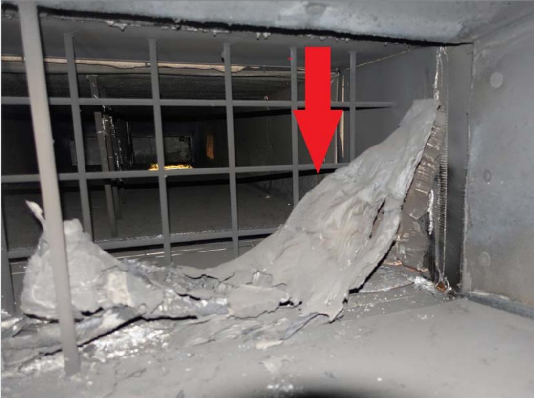
Figure 4. Charred Cardboard Left in the Ductwork
