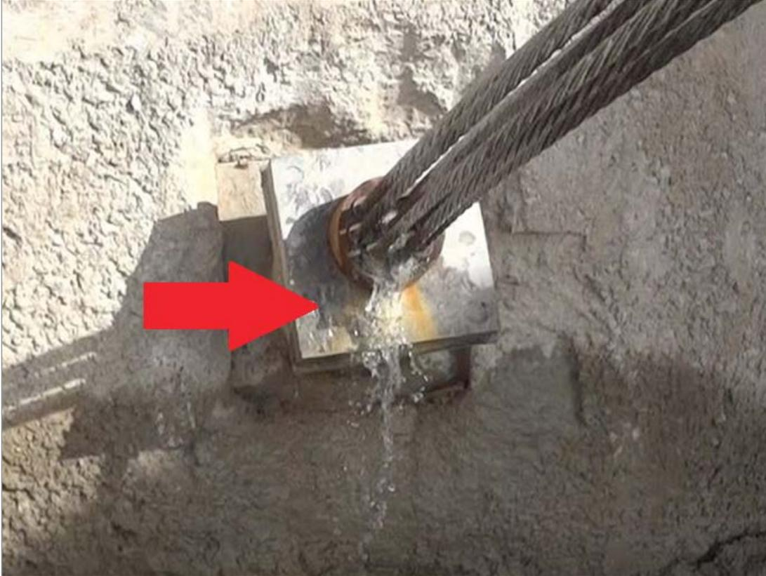
Figure 2. Water Leaking from the PERS Wall
