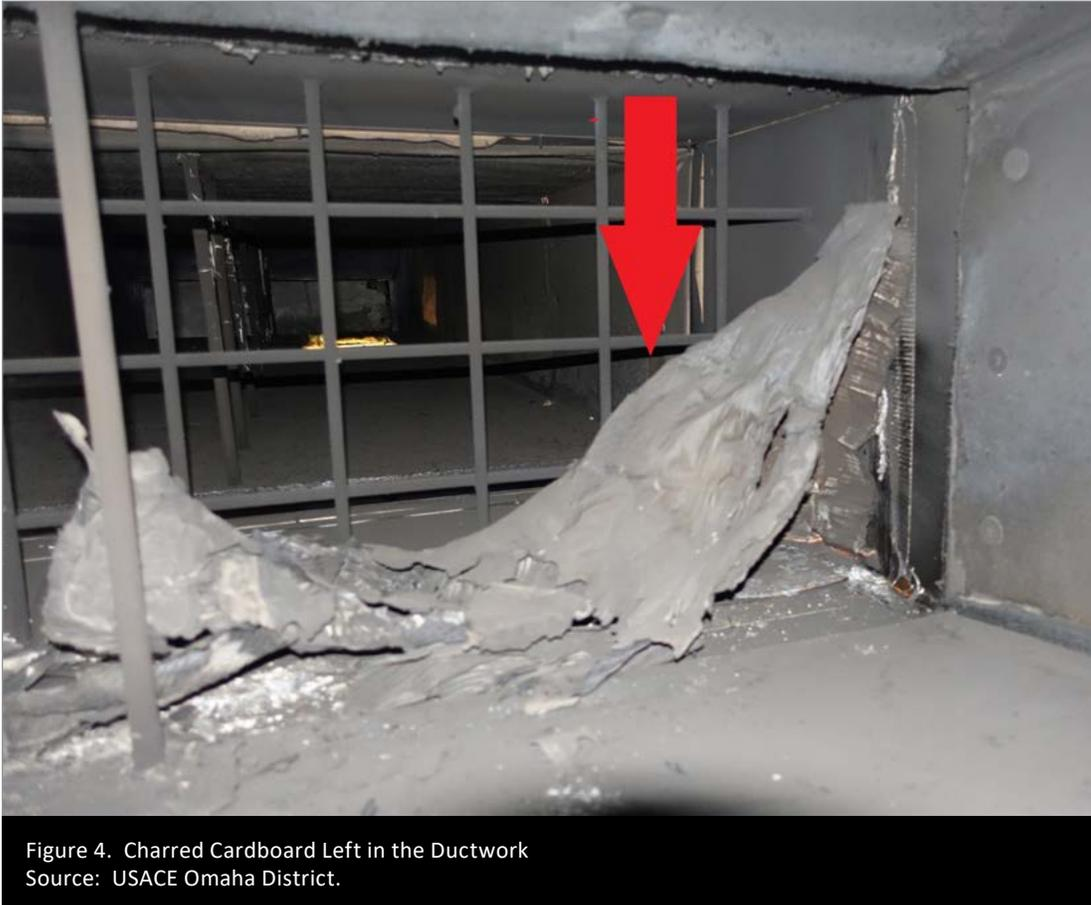
Figure 4. Charred Cardboard Left in the Ductwork
