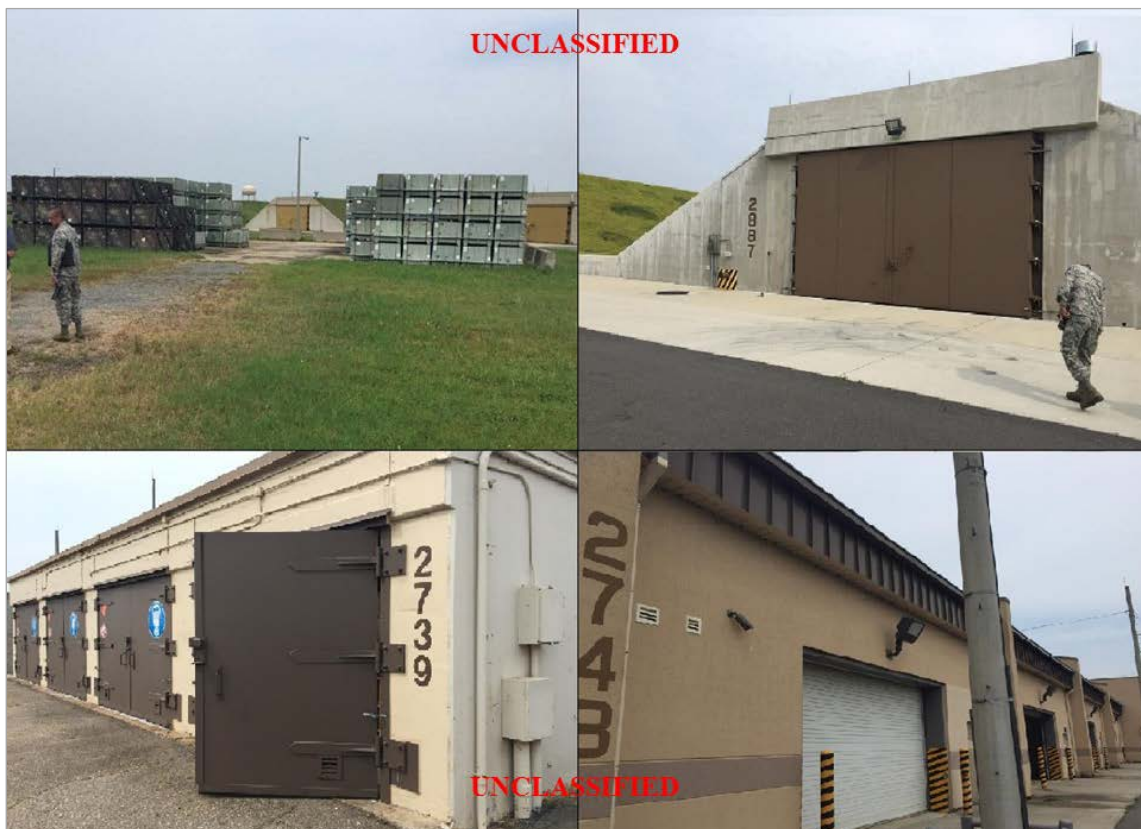
(U) Figure 1. Open-Area Storage, Earth-Covered Magazine, Operating Location, Multi-Cube Building. (Clockwise, From Top-Left)
