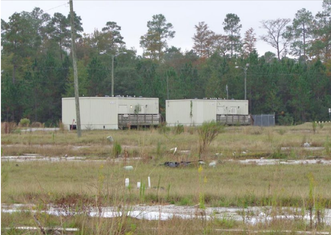
Figure 4. Field on Fort Stewart Where Relocatable Buildings Were Removed Source: DoD OIG.
