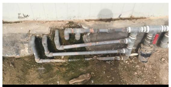
Figure 6. Water Leaks in the Delta Block Source: DoD OIG
