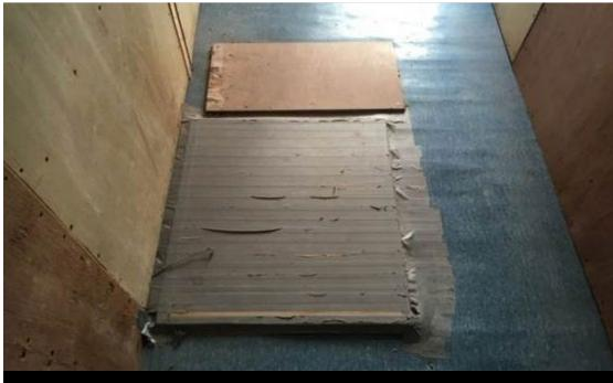
Figure 5. Temporary Patch for Holes in Housing Unit Floors Source: DoD OIG
