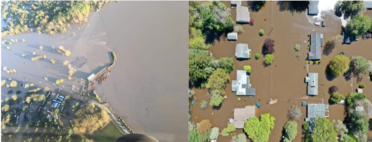
Figure 2 (left). Image of the failed Sanford Dam in Michigan Figure 3 (right). Several homes inundated under floodwaters in Midland, Michigan
