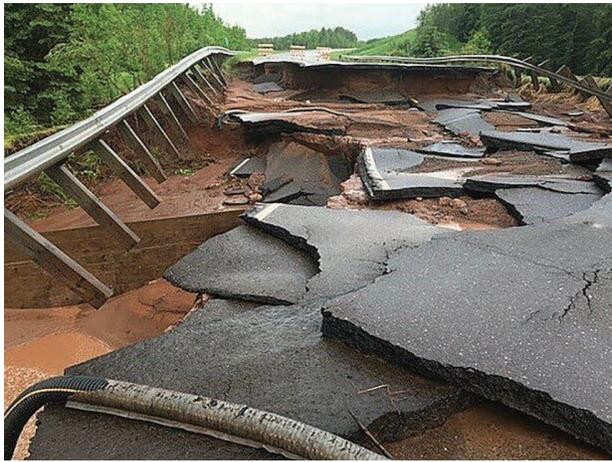
**Figure 3.** Damage caused by flash flooding on State Highway 23, Carlton County, MN
