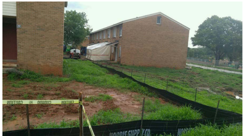
Figure 3 – Encapsulated remediation of asbestos, 310 Highland Ave., Spartanburg, SC.
