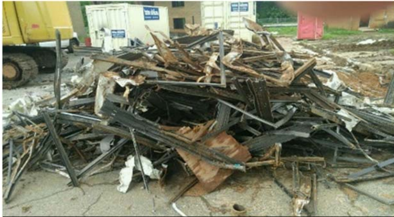
Figure 6 – Aluminum scrap pile recovered from the razing of 331 S. Forest St.
