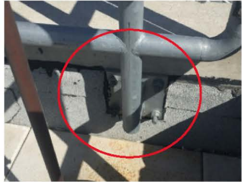
Figure 6: Improper installation of roofing on sidewall. Source: Photograph taken by OIG in April 2019.
