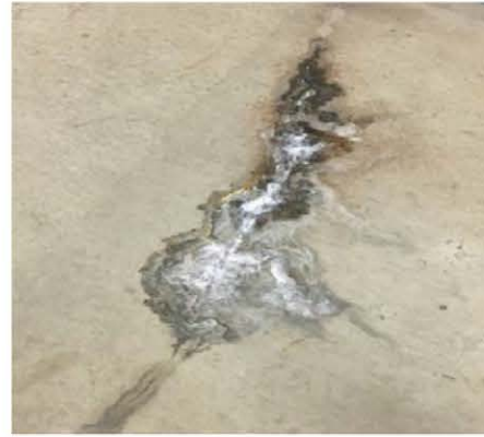
Figure 3: Ground water seeping through the lower level floor of NEC London. Source: OIG photograph taken January 2020.
