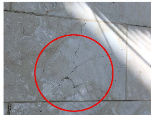
Figure 9: Damaged (cracked) interior stone tiles. Source: Photograph taken by OIG in April 2019.
