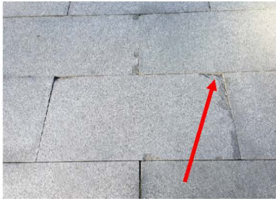
Figure 10: Damaged edges of exterior stone pavers on embassy driveway.
