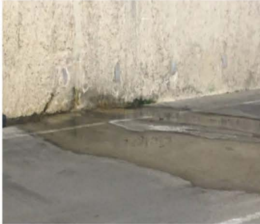
Figure 2: Ground water seeping into the lower level parking garage of NEC London. Source: OIG photograph taken January 2020.
