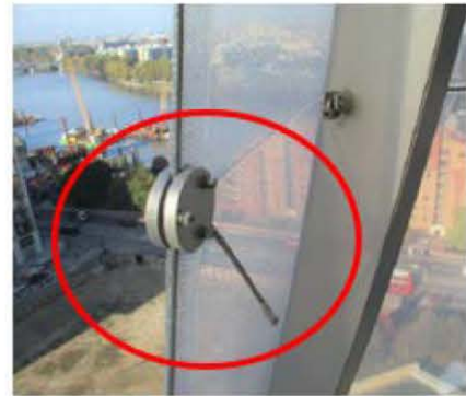
Figure 7: Wind Cable detached from building. Source: Photograph from Stan Ltd. Inspection.
