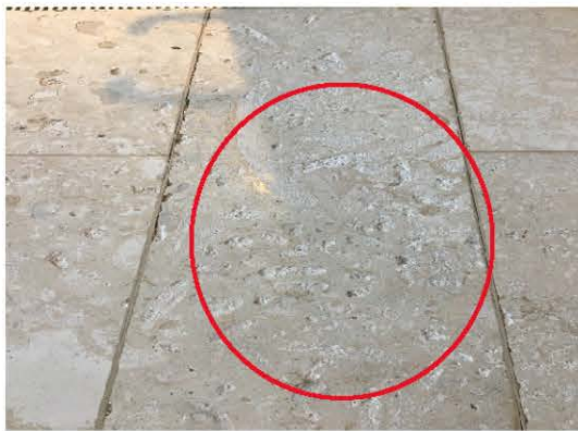
Figure 8: Damaged interior stone tiles on sixth floor showing spalling and delamination. Source: Photograph taken by OIG in January 2020.
