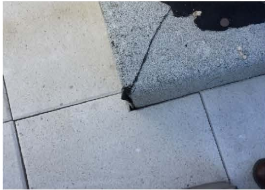
Figure 5: Improper installation of roofing over equipment pad. Source: Photograph taken by OIG in April 2019.
