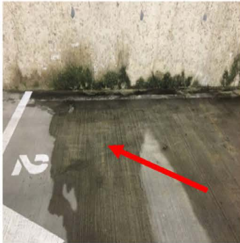
Figure 4: Mold forming on the wall in the lower level parking garage of NEC London. Source: OIG photograph taken January 2020.
