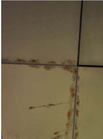
Figure 3: Stainless-steel panels under the eaves of the Main Compound Access Control facility at Embassy The Hague.
