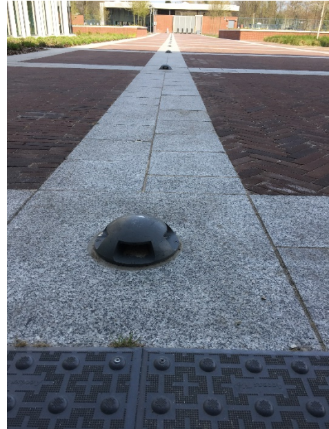
Figure 2: Raised lights separating walkway from driveway at Embassy The Hague. Source: OIG photograph taken April 2019.
