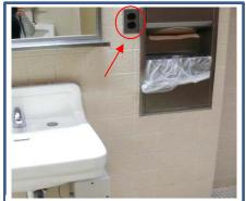
Figure 4: The circled electric receptacle between the sink and the towel dispenser is not ground fault circuit interrupter protected.
