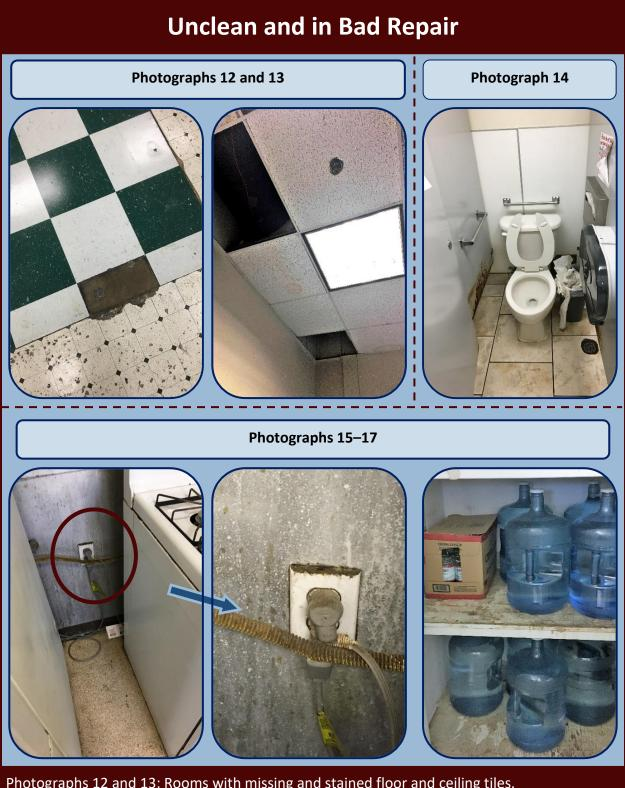
Photographs 12 and 13: Rooms with missing and stained floor and ceiling tiles. Photograph 14: Restroom with overflowing trash cans and rust on stall partitions. Photograph 15 17: Kitchen with dirt buildup on gasline and electric outlet and dirty cupboards.
