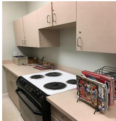
Photograph 6 (left): Functioning stove without installed class K fire extinguisher. Photograph 7 (right): Obstructed sprinkler head in resident room closet.
