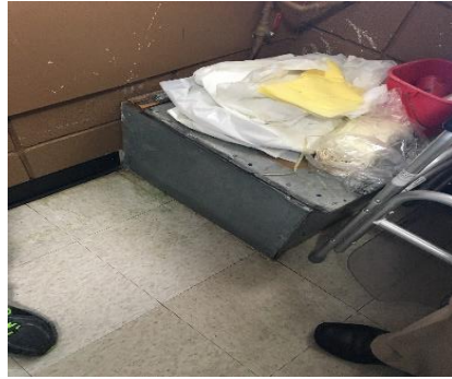
Photograph 1 (left): Top of unused laundry chute not sealed with fire caulk. Photograph 2 (right): Unsealed bottom of unused laundry chute.
