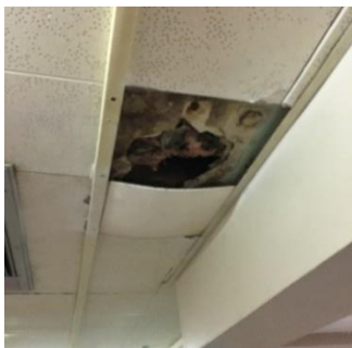
Photograph 3 (left): Ceiling smoke/fire barrier in facility hallway in disrepair. Photograph 4 (center): Battery backup for emergency lighting not working. Photograph 5 (right): Exit discharge lighting missing bulb.
