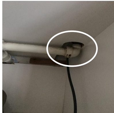
Photograph 6 (left): Functioning stove without installed class K fire extinguisher. Photograph 7 (right): Obstructed sprinkler head in resident room closet.
