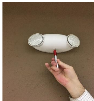
Photograph 3 (left): Ceiling smoke/fire barrier in facility hallway in disrepair. Photograph 4 (center): Battery backup for emergency lighting not working. Photograph 5 (right): Exit discharge lighting missing bulb.
