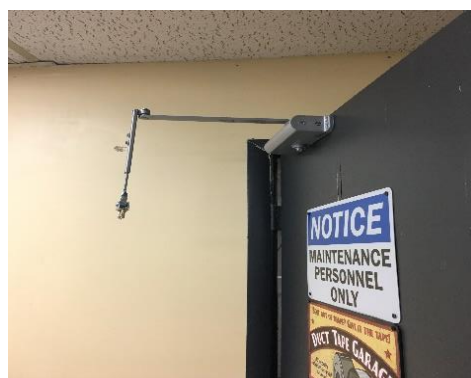
Photograph 8 (left): Hazardous area enclosure’s self-closing device not closing properly. Photograph 9 (right): Hazardous area enclosure’s self-closing device disconnected.
