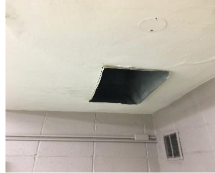
Photograph 1 (left): Top of unused laundry chute not sealed with fire caulk. Photograph 2 (right): Unsealed bottom of unused laundry chute.
