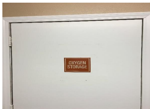
Photograph 10 (left): Unsecured gasoline cans not stored in a flammables storage cabinet. Photograph 11 (right): Oxygen storage room lacking a posted “NO SMOKING” sign or symbol.
