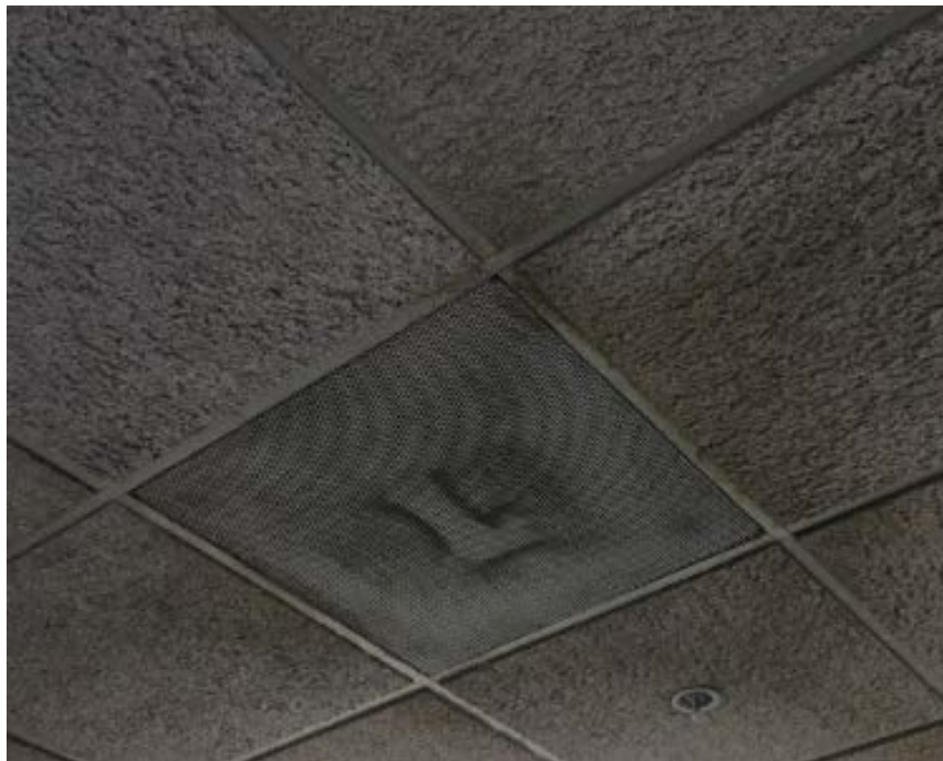
Figure 7: Discolored Ceiling Tiles in Facility Hallway
