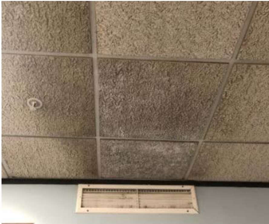
Figure 8: Discolored Ceiling Tiles in Facility
