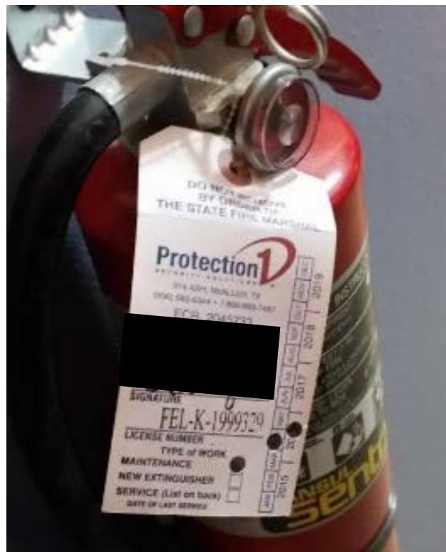
Figure 15: Fire Extinguisher With Expired Inspection Tag Located in Hallway of UAC Living Space (Photo Taken in September 2017)
