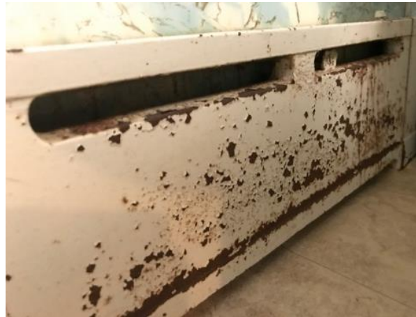
Photograph 16: Rust covered a bathroom radiator (WI).
