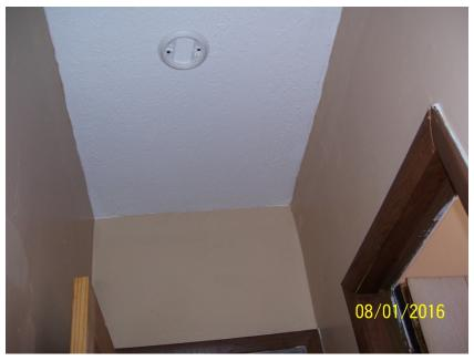
Photograph 12: A smoke detector was missing.
