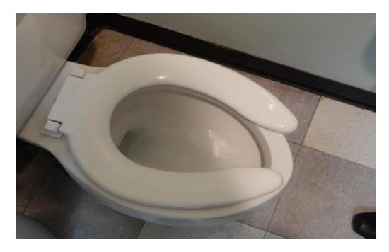
Photograph 6: This toilet seat was not fastened to the toilet and could be a hazard.
