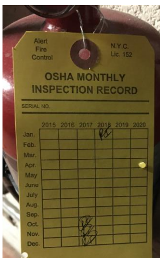
Photograph 6: Fire extinguisher did not have February and March 2018 inspections documented. New annual tag attached in October 2017. Photograph taken on April 4, 2018.
