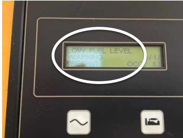
Photograph 15: Generator fuel gauge indicating low fuel level warning.
