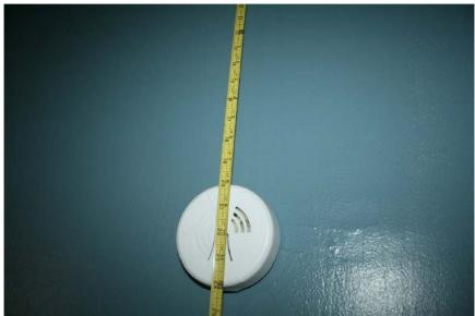
Inspection 71: The smoke detector was not properly mounted. Smoke detectors should be no less than 4 inches from the ceiling but no more than 12 inches from the ceiling. It was 20 inches from the ceiling. The Authority did not identify this violation during its May 18, 2017, inspection.
