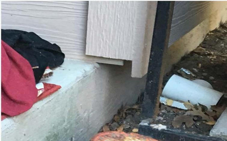
The frame of the house extended over the slab by inches.
