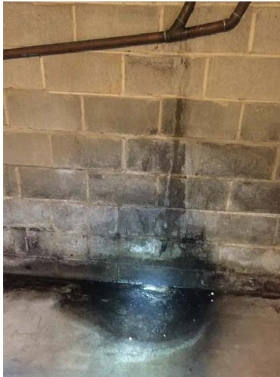
Inspection 34: A drain in the basement leaked on the wall and floor. The Authority did not identify this violation during its January 18, 2017, inspection.
