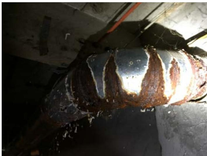
Inspection 60: A corroded furnace flue had holes in it. The Authority did not identify this violation during its November 1, 2016, inspection.
