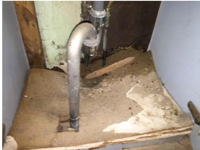
Inspection 51: The floor in the basement bathroom vanity was moisture damaged and collapsed. The Authority did not identify this violation during its November 28, 2016, inspection.
