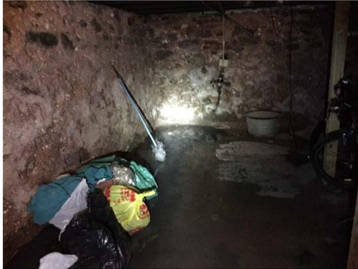
Inspection 11: The foundation walls leaked, leaving puddles and silt on the basement floor. The Authority did not identify this violation during its January 12, 2017, inspection.
