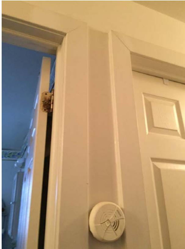
Inspection 38: The smoke detector in the 2<sup>nd</sup> floor hall was installed too low on the wall. The Authority did not identify this violation during its November 14, 2016, inspection.
