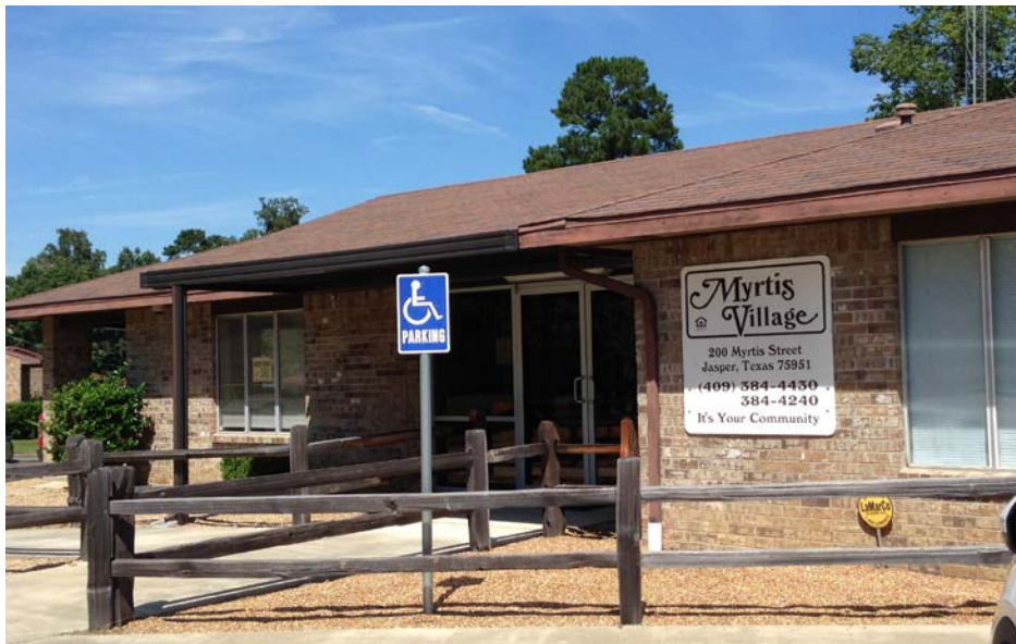
Figure 1: Main office of the Housing Authority of the City of Jasper, TX
