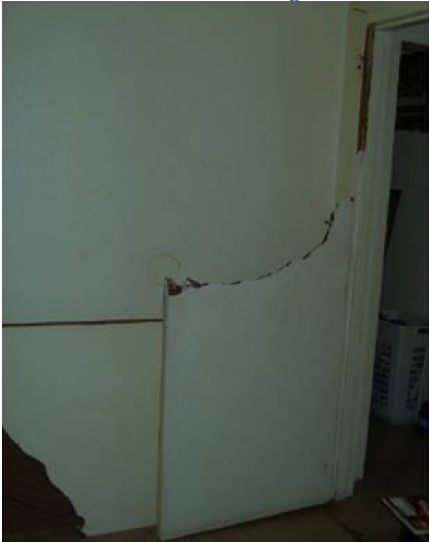
Behner Place unit, 4112 36th Street
