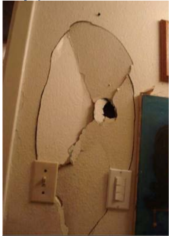
Behner Place unit, 4109 35th Street
