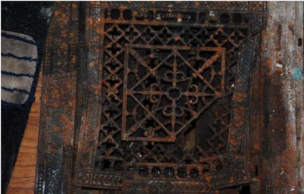
The picture above shows a damaged cast iron grill on an air vent on the bathroom floor.
