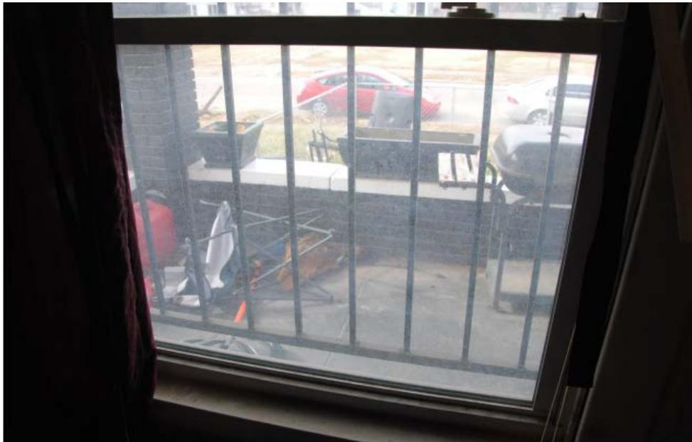
The picture above shows bars on a front bedroom window, which block the tenant's ability to exit the room in case of an emergency.
