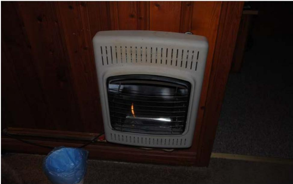
The picture above shows a ventless, open-flame heater mounted on the living room wall, which creates a health and safety hazard.
