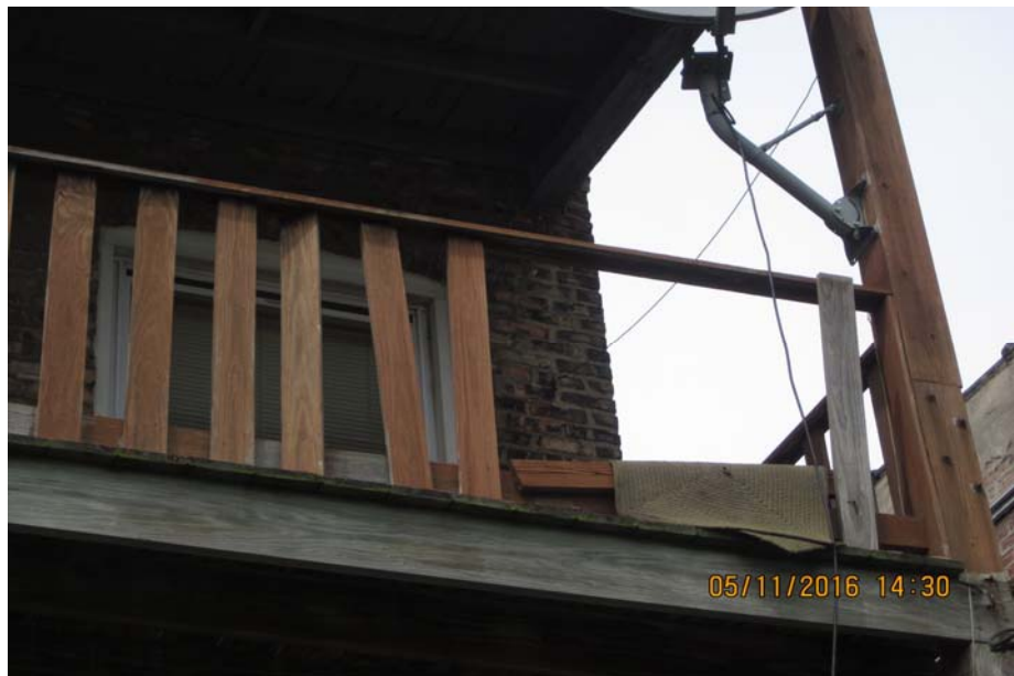
Property #A123: Missing midrails (balusters) on second floor
