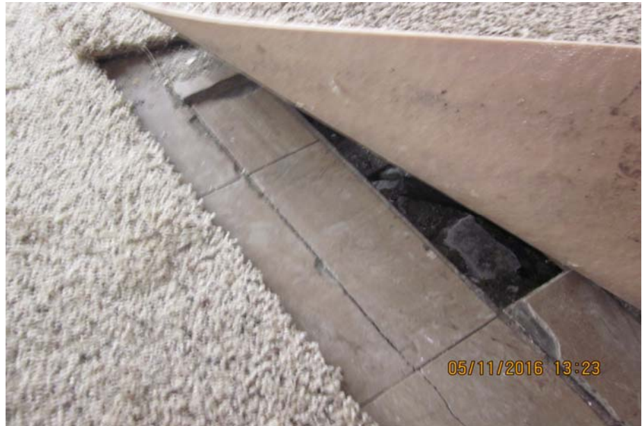
Property #A122: Missing flooring covered up with carpet
