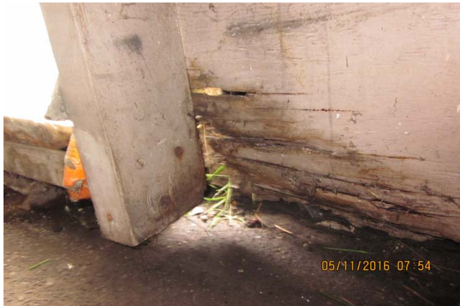
Property #A117: Deteriorated basement wall
