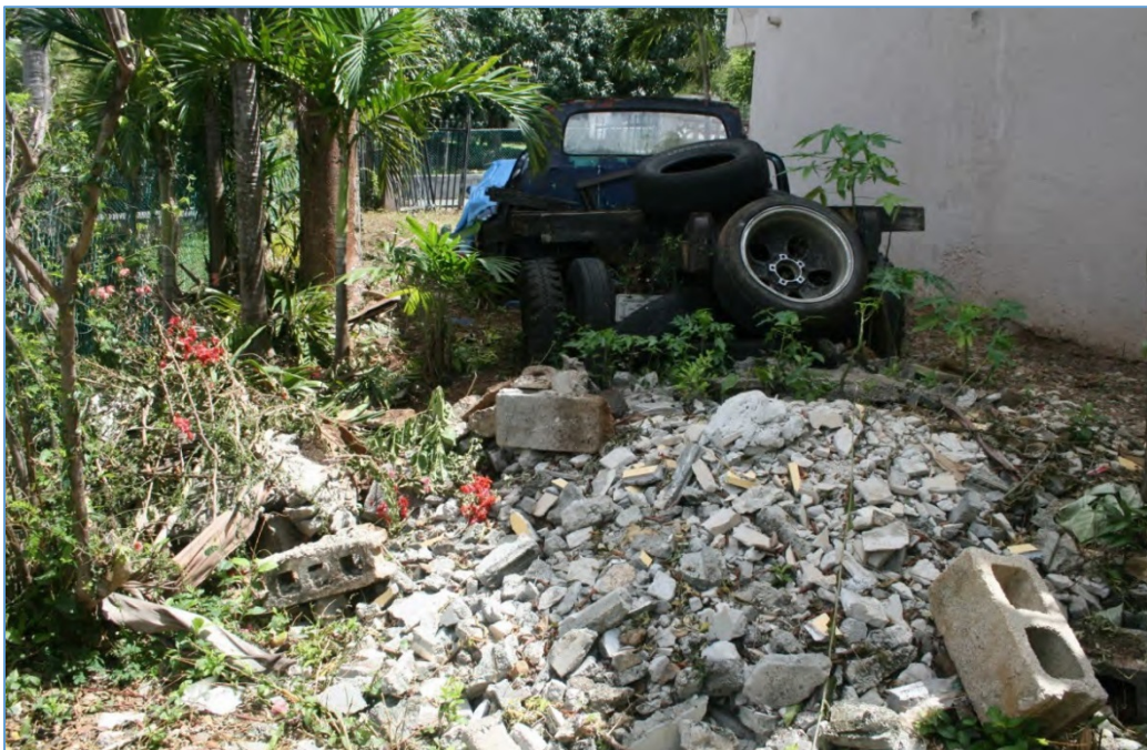
The picture above shows abandoned vehicles, concrete blocks, and construction debris piled up in the yard of unit. This clutter does not promote safe and sanitary conditions.
