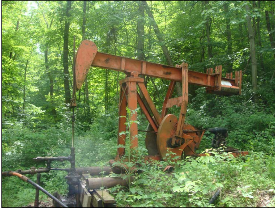
Figure 2. This pump jack is located near a hiking trail in the Wayne National Forest. Source: OIG.
