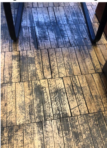
Figure 5. Worn Flooring
