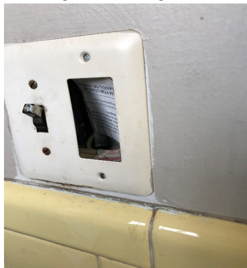
Figure 13. Missing Outlet
