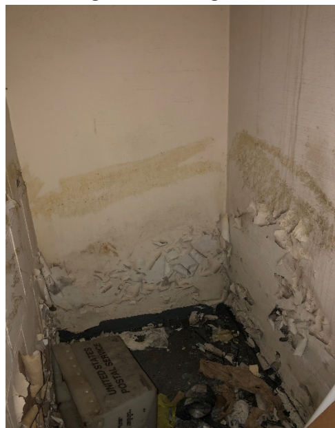
Figure 2. Peeling Walls
