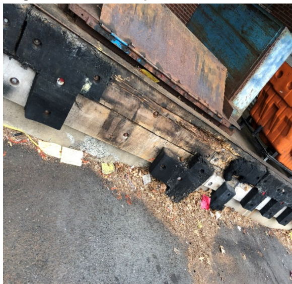
Figure 4. Trash, Bumpers, and Rotted Wood
