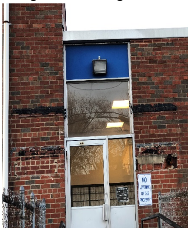
Figure 6. Missing Bricks
