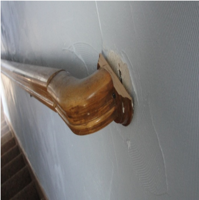
Photographs 6 and 7: Staircase with a broken handrail and broken balusters, which weakened the banister/railing system.
