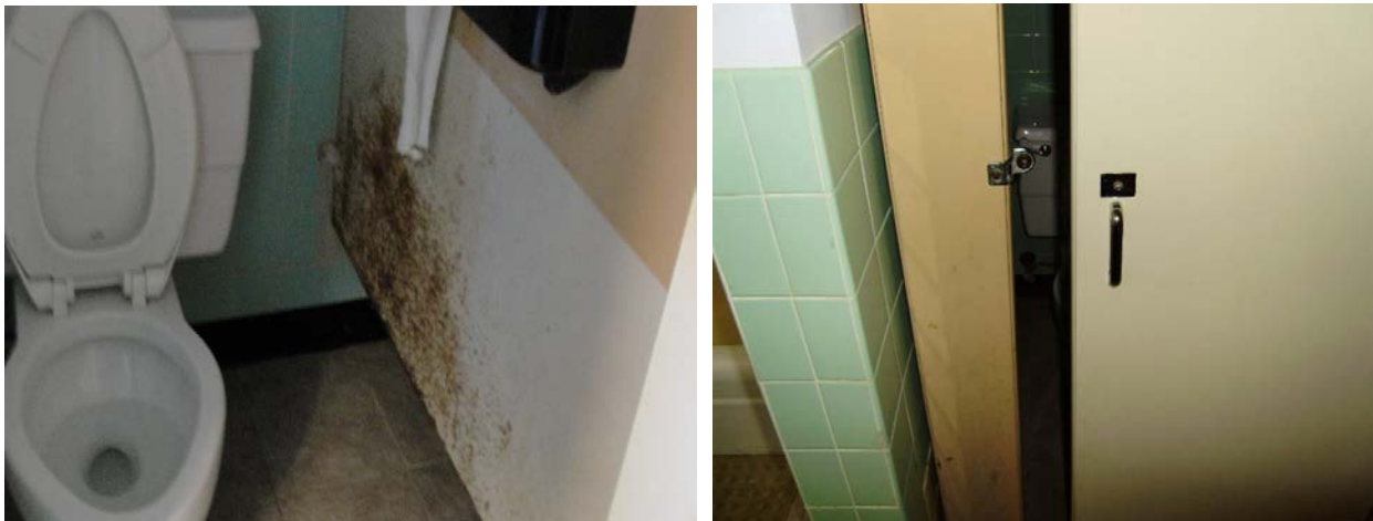
Photographs 17 and 18: Rusty bathroom stall walls and a bathroom stall door that did not fit properly, preventing user from having full privacy.
