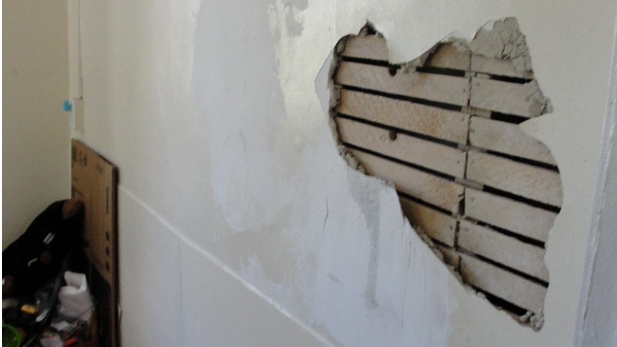
Photograph 8: A hole in a bedroom wall exposing the wall's frame.
