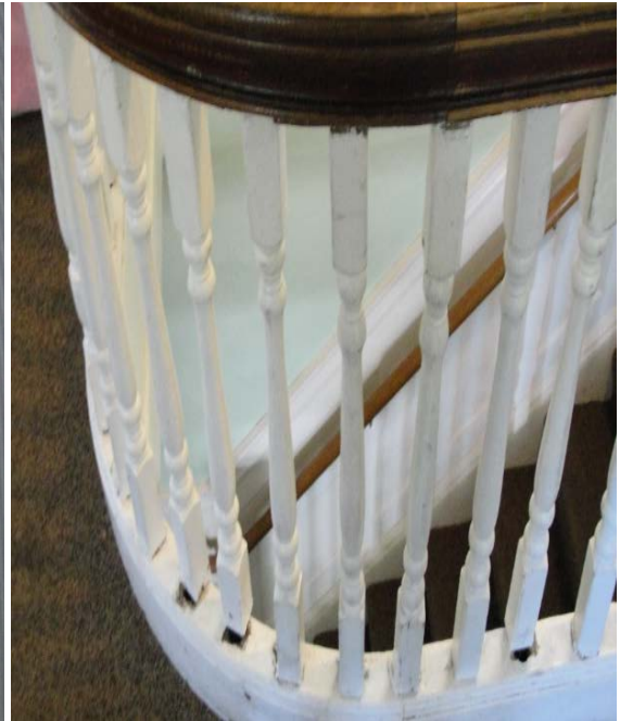
Photographs 6 and 7: Staircase with a broken handrail and broken balusters, which weakened the banister/railing system.
