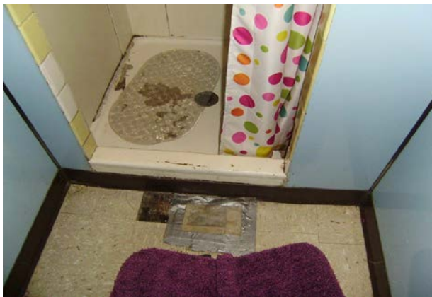
Photograph 14 and 15: Water-damaged bathroom floor, dirty shower mat, a shower with mildew within the tile crevices, and a moldy shower curtain.
