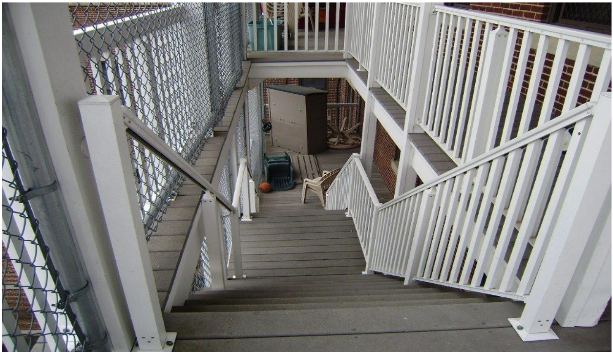
Photograph 20: Looking down the fourth-floor staircase of outdoor porch, which did not have a barrier to protect younger children from a potential falling hazard.
