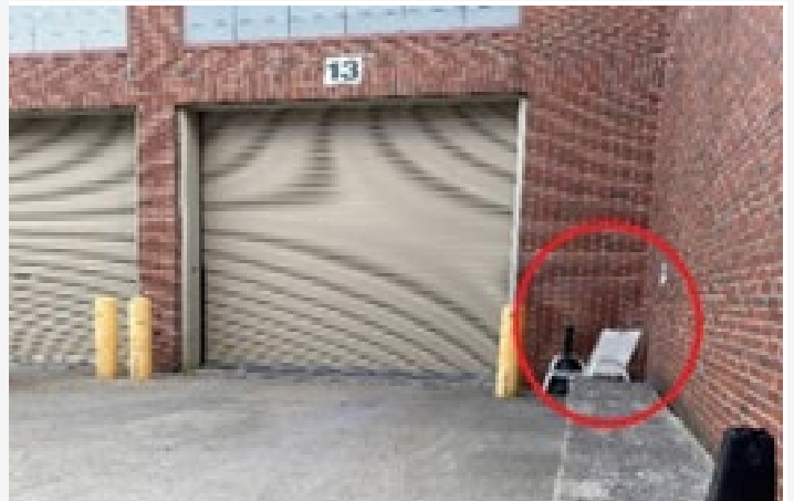
Source: Site visit to Boston VMF on May 25, 2023.
