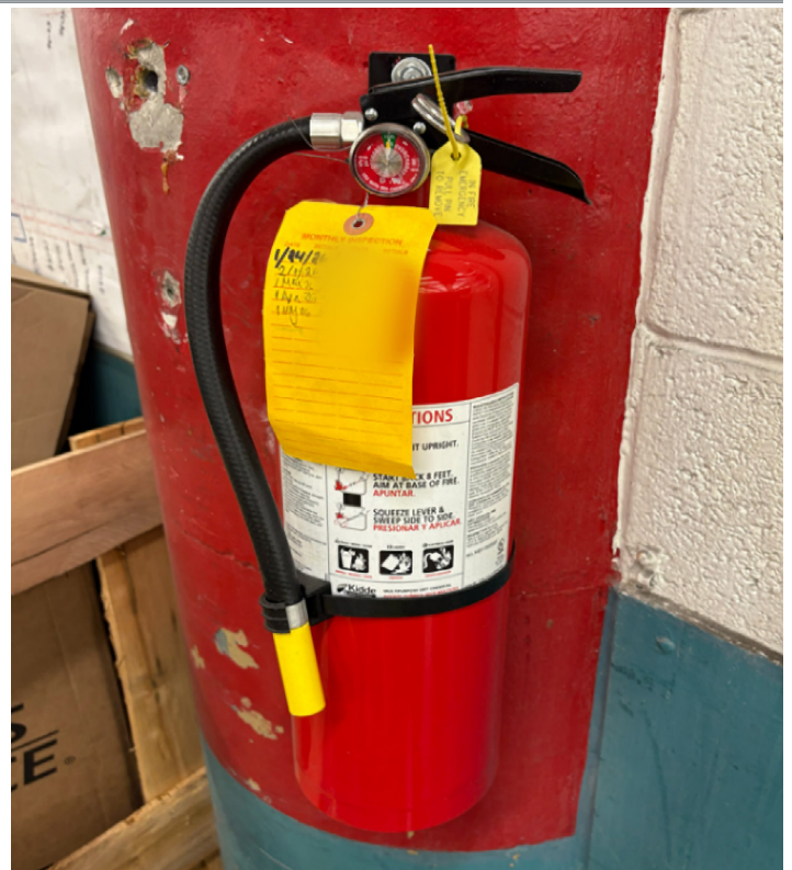
Figure 2. Fire Extinguishers With Expired Inspection and No Annual Inspection Tag
