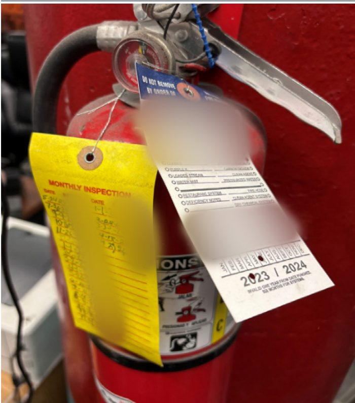
Figure 2. Fire Extinguishers With Expired Inspection and No Annual Inspection Tag
