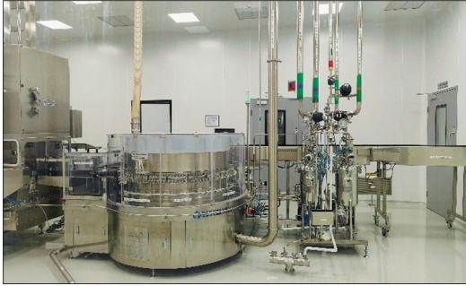
Image of Bio E pharmaceutical manufacturing Facility
