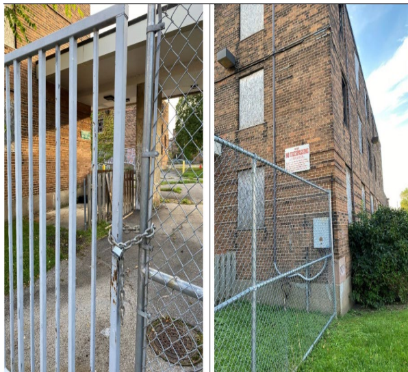
Figure 5. Entire development was vacant and uninhabitable
