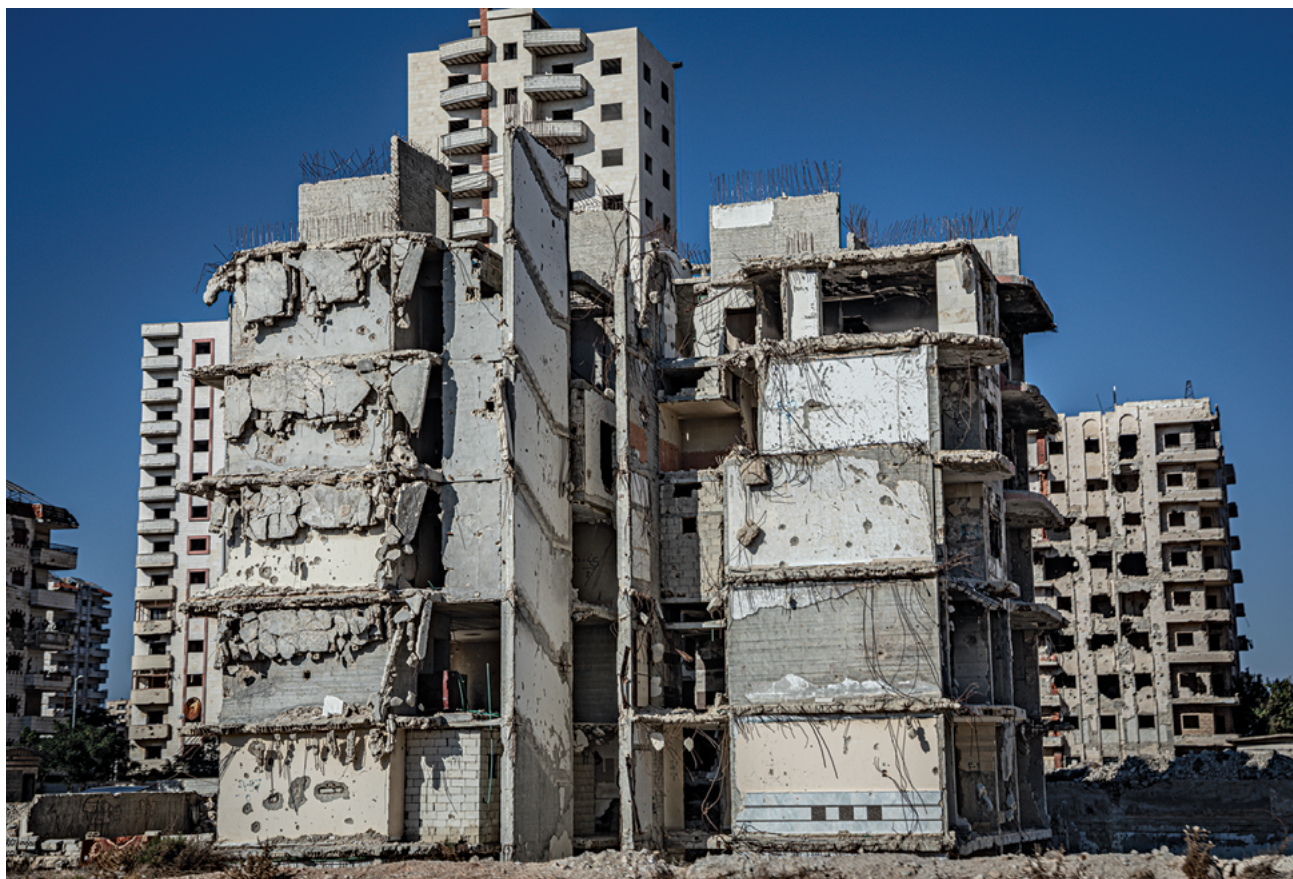
Damaged and destroyed buildings in Homs, Syria. (UNHCR photo)
