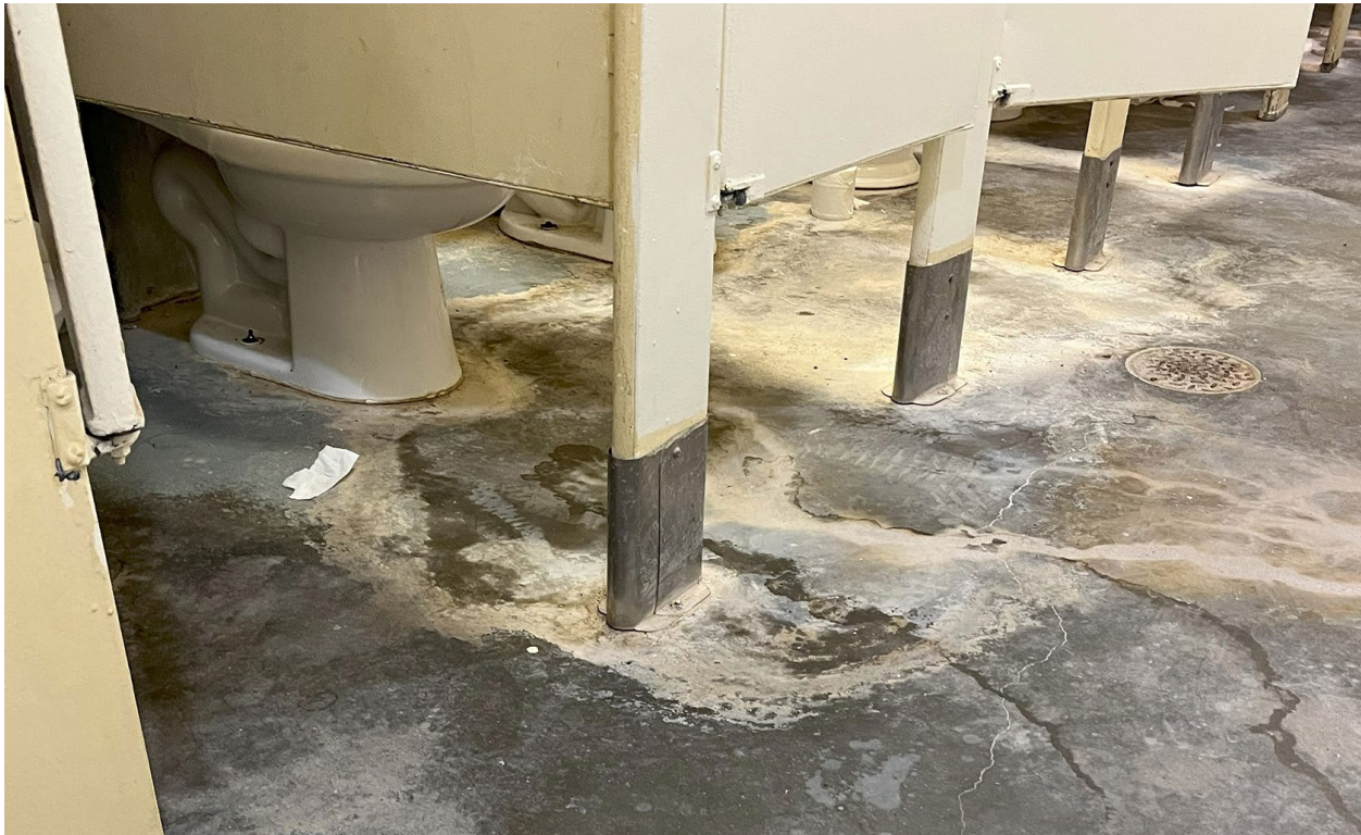
Figure 2. Dried Raw Sewage on the Floor of a Bathroom at the Doña Ana Range Complex in Chaparral, NM, Observed on July 27, 2025 Source: The DoD OIG.
