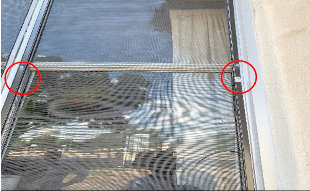
Figure 3. Screen Screwed into Window Frame at Randolph Air Force Base in Universal City, TX, Observed on June 13, 2024 Source: The DoD OIG.
